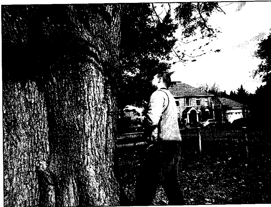
Photo 12. Determining depth of cavity on south side of T1.
