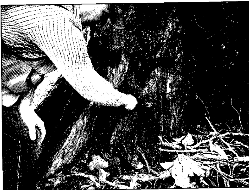
Photo 20. Probing crack at base of T2 to determine depth of cavity inside.
