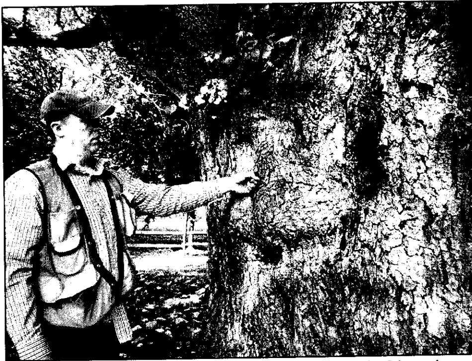
Photo 22. Probing cavity on west side of T2 to determine depth of the cavity.
